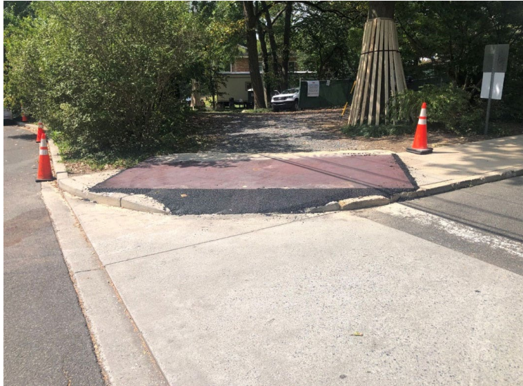
Re-installed Construction Entrance at Fletcher Gate at American University
