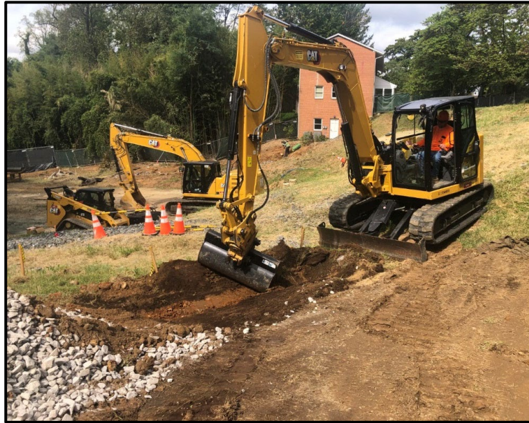
Excavating Eastern Drainage Swale for erosion control
